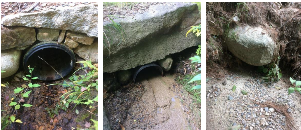
Figure 5: Examples of various amounts of sediment build up in Tuftonboro, NH.
