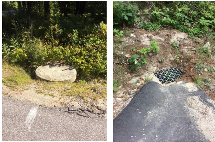
Figure 2: Examples of 'Catch Basin Inlets' in Tuftonboro, NH. (Left: County Road, Right: Sodom Road)
