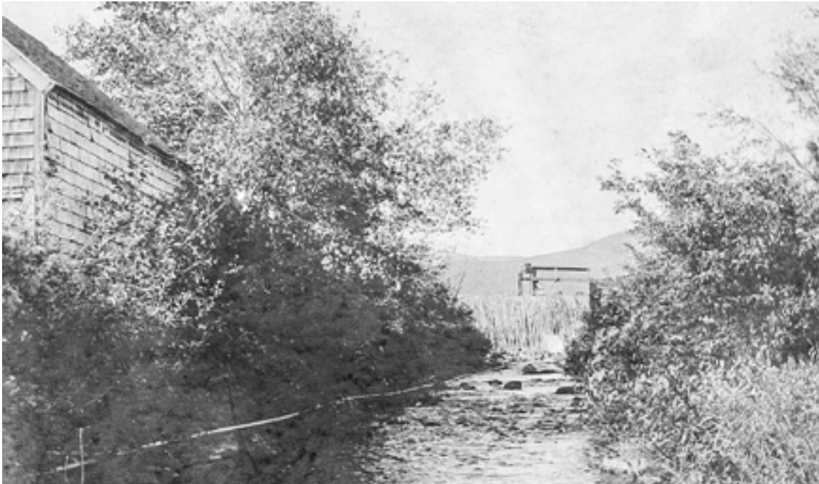
The Boody grist mill and dam on the Melvin River, circa 1900. The dam was constructed of logs, earth and rocks and was located at the present site of the Pope Dam in Melvin Village. Built in 1850, the earthen dam eventually disintegrated. The Pope Dam was built in 1952. Photo courtesy of the Tuftonboro Historical Society.
