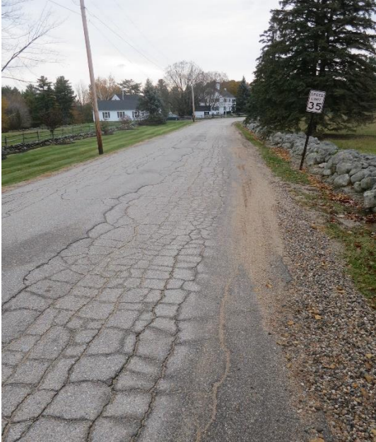
An example of Alligator Cracking on North Line Road
