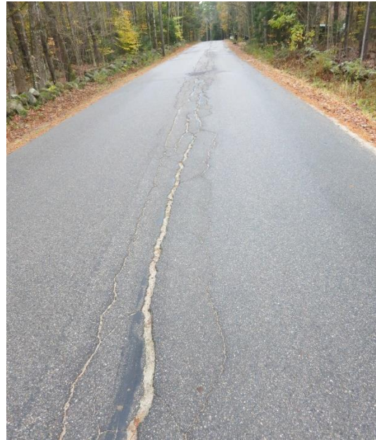
An example of Longitudinal Cracking on Dame Road
